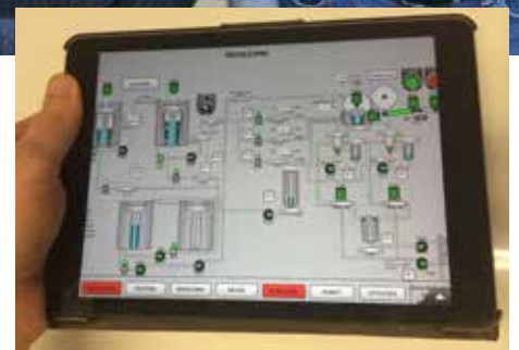
SCADA Screen displayed on the iPad
